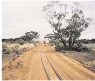
Cables laid-out prior to burying.
