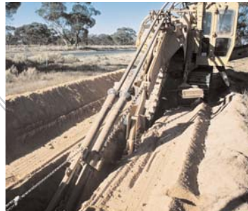
Purpose built machines cut channels causing minimal disturbance.
